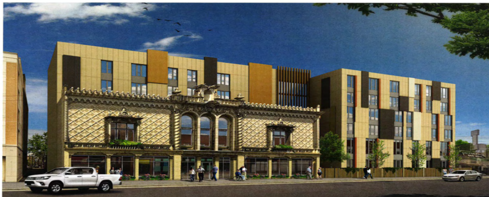
1535 North Pulaski Road 61 Affordable-Elderly Apartments in West Humboldt Park
